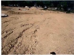
Photo Taken: 4/13/2021 10:10:18 AM Erosion rills and gullies were observed on slopes.
