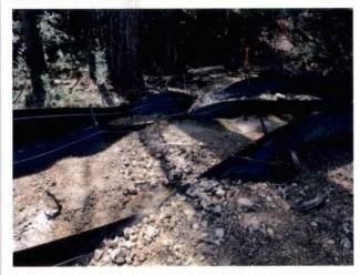
Photo Taken: 4/13/2021 10:01:41 AM Excessive sediment accumulation was noted at silt fencing.
